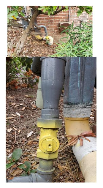
The valve is YELLOW for quick identification. As with the water valve, When the handle is verticle as seen in the photo the gas is on, when the handle is horizontal the gas is off. Because it is a gas valve a tool is needed to shut it off. The tool is located (WHERE DO YOU WANT TO KEEP THIS TOOL?)
